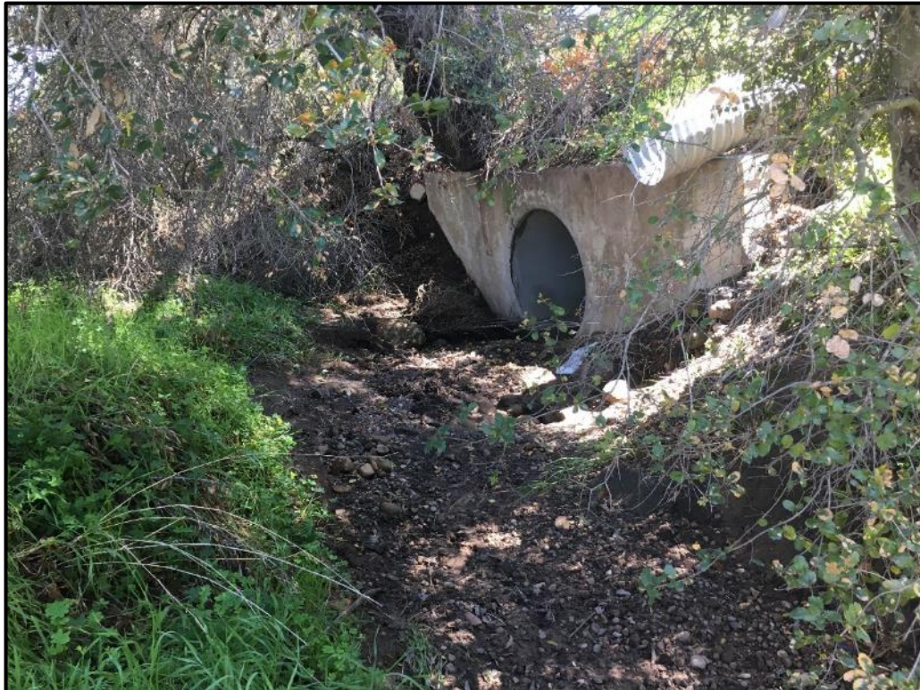
Photo 4. Culvert at the south end of the drainage that conveys runoff under Calle Real and Hwy 101 to Hospital Creek (Aspect: Southeast). Photo taken March 23, 2018.
