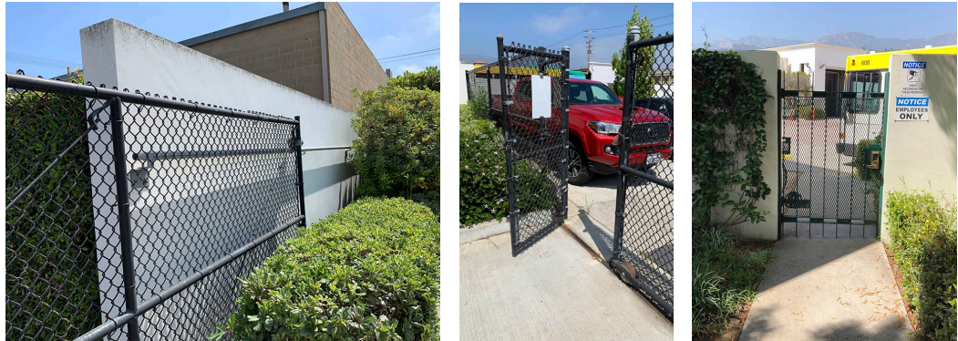
Mid-Parking Lot vehicle Rolling Gate and Staff Gate / Staff Gate Directly to the Bus Yard
