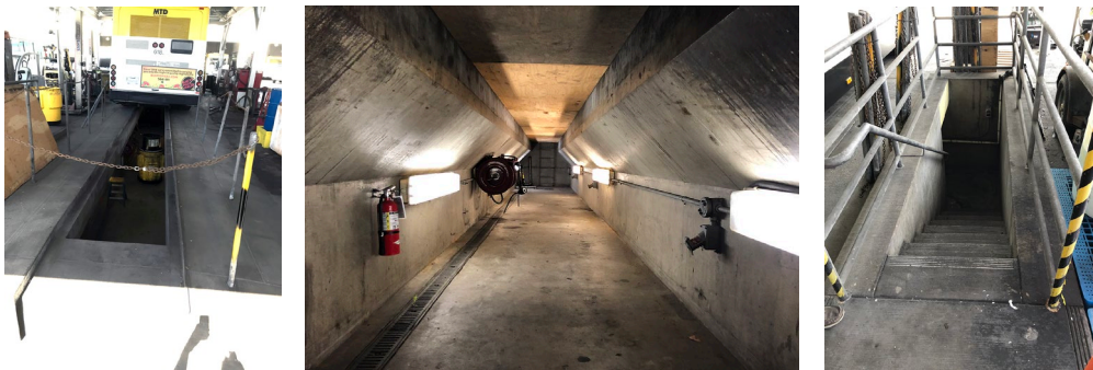
Service & Inspection Pit: Pit Opening w/ Guard Posts / Pit w/ Lighting / Stair Down to Pit
