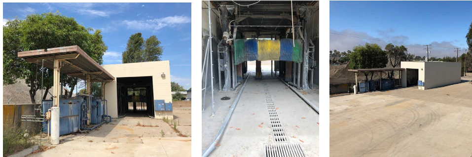
Equipment Canopy / Wash Bay Interior / Bus Wash Building
