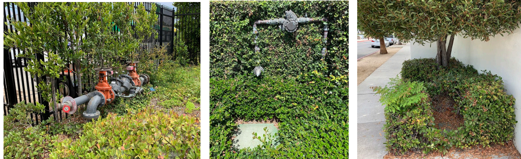
FDC Next to Administration Building | Buried Utility Connections
