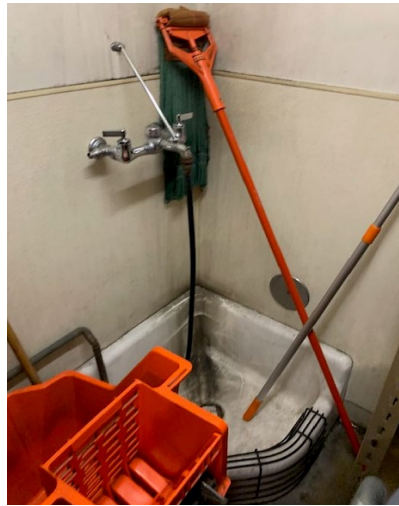
Figure 9: Janitor Sink and Faucet Figure 10: Drain w/ Proper Protection
