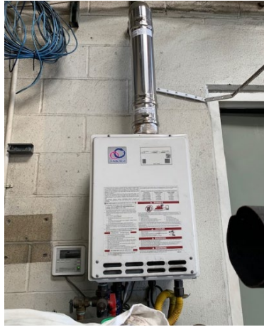
Figure 15: Tankless Water Heater
