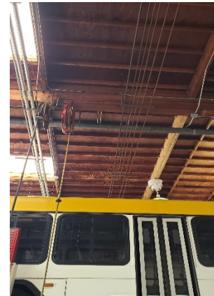
Figure S-2: Repaired Wood Framing
