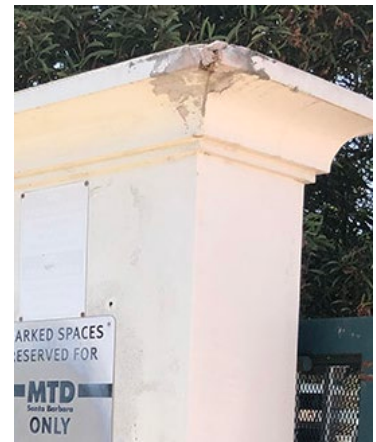
Haley St Rolling Gate / Latch End of Gate / Chipped Site Fence Cornice in Need of Repair
