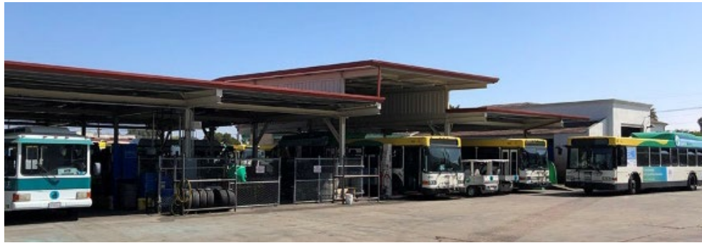
View from Maintenance Garage to Center Canopy
