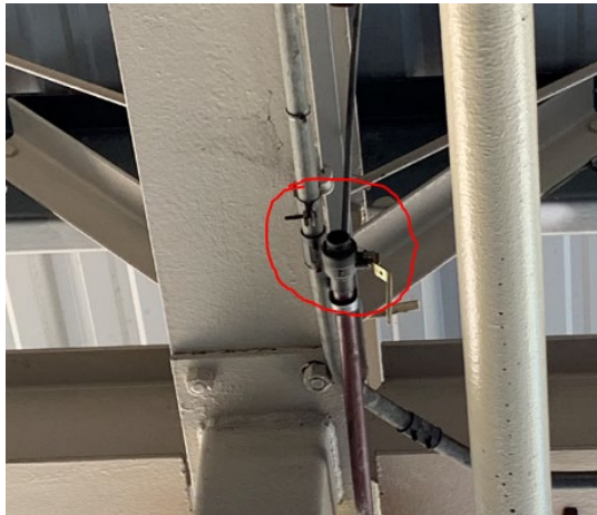
Open Ended Pipe in the Service Pit
