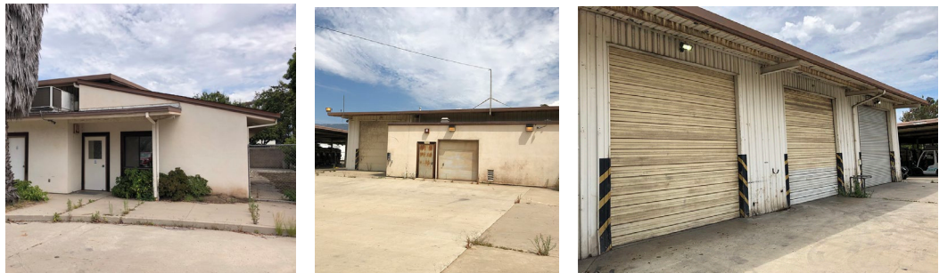
Exterior of Terminal 2 Maintenance Building
