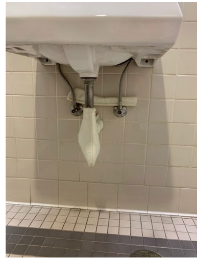
Figure 9: Janitor Sink and Faucet Figure 10: Drain w/ Proper Protection
