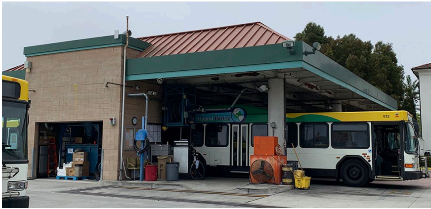
View from Front Yard to Fuel Island
