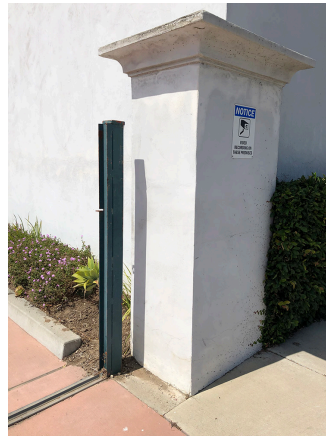
Haley St Rolling Gate / Latch End of Gate / Chipped Site Fence Cornice in Need of Repair
