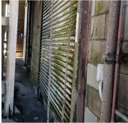
Figure S-7: Bus Wash Metal Coil Door
