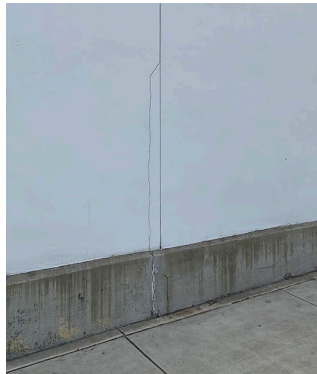
Wall Crack Showing Settlement / Anti-Graffiti-Coating | Exit Door
