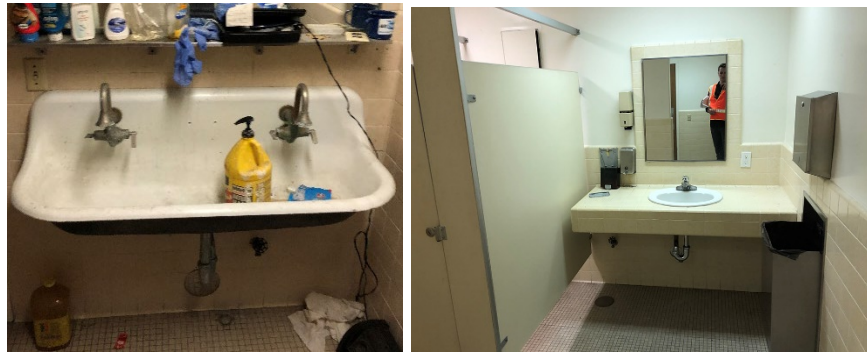
Maintenance Restroom Handwash Basin / Women's Restroom
