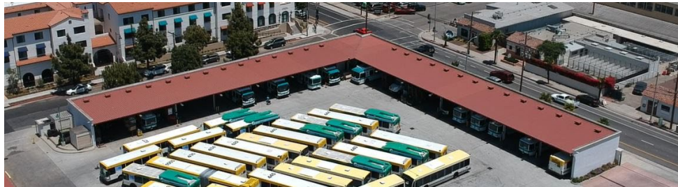
Electric Bus Canopy Aerial Photo
