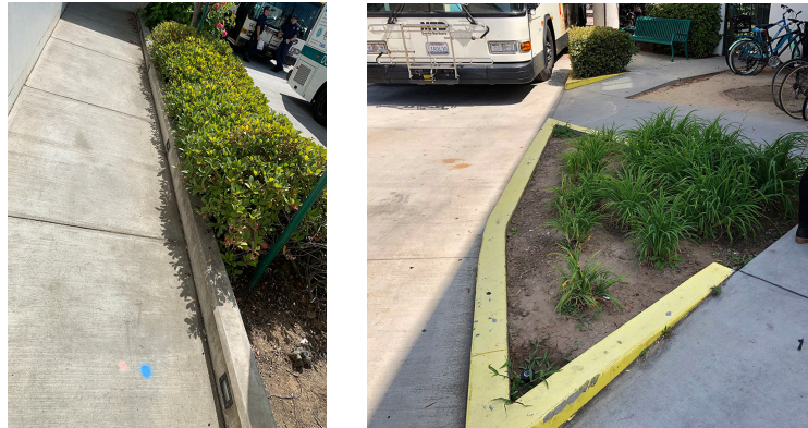
Footpath Lighting at North Ramp of Admin Building / Planted Area at Staff Entry/Exit from Admin Building into the Bus Yard
