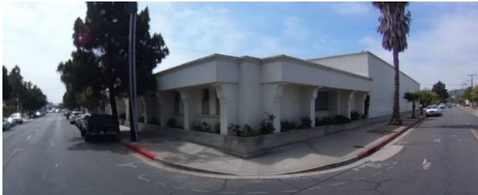
Maintenance Garage/Shop corner at Salsipuedes St. and Cota St.
