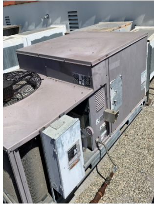
Figure 1: Carrier Package Heat Pump Units
