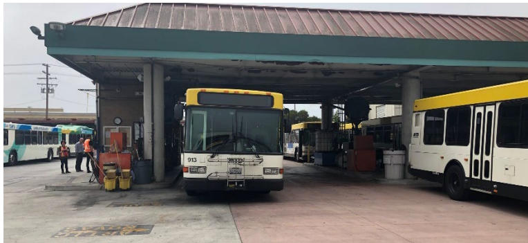
The two fuel-service islands at Terminal 1
