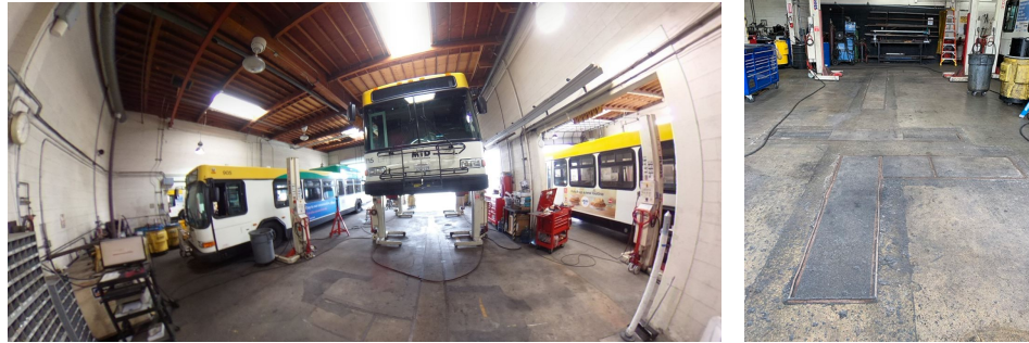
Typical Maintenance Bay | Abandoned In-Place Lift with Concrete Fill
