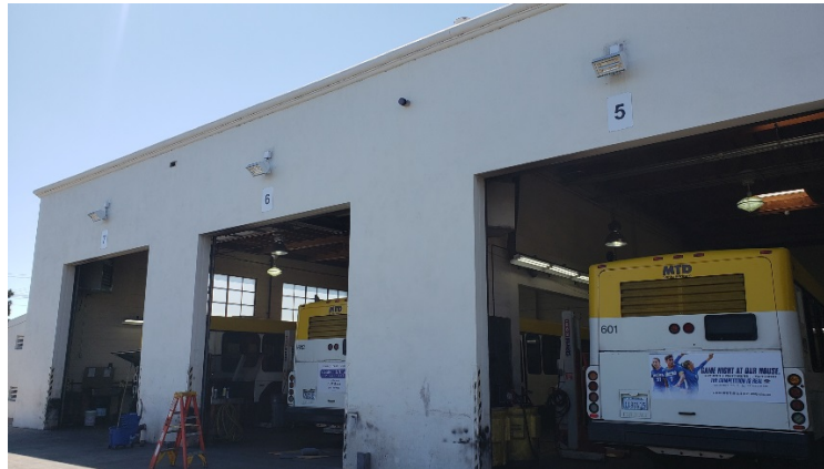
Floodlights and Interior Pendant HID
