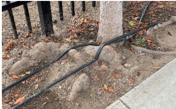
Tree Roots pinching irrigation lines / Typical fencing on Olive St and Cota St – gate shown here, only opened to access the SCE vault below.
