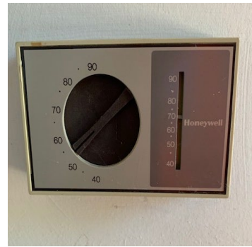
Figure 6: Elevator Room Thermostat w/ No Supply
