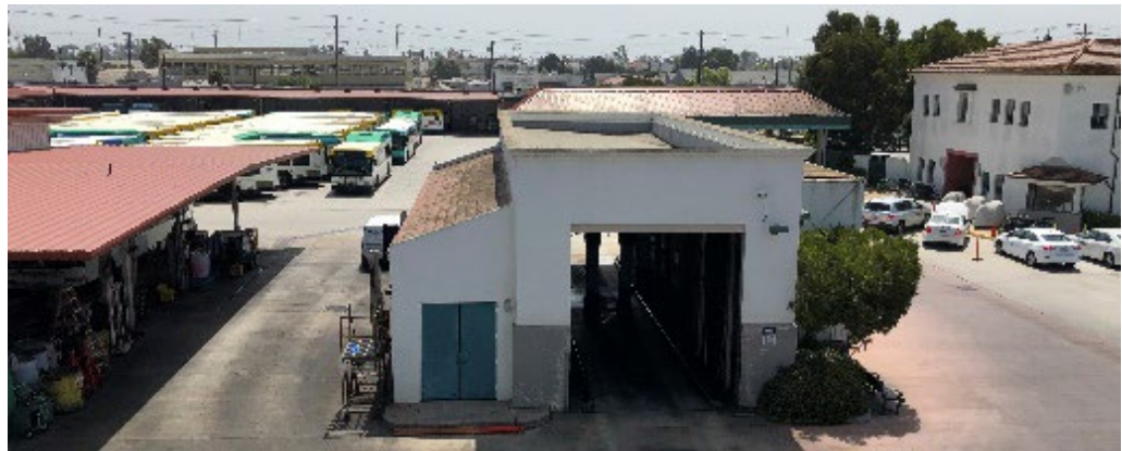
Wash Bay Building (looking south)
